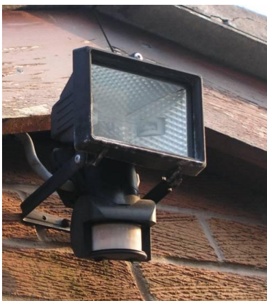
Passive Infra-Red detector mounted below a 300W Tungsten Halogen Fitting
