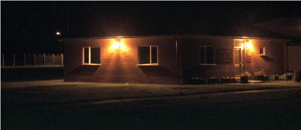
Building walls illuminated using 70 W SON in bulkhead fittings.
