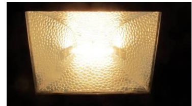
TH Lamp in a luminaire
