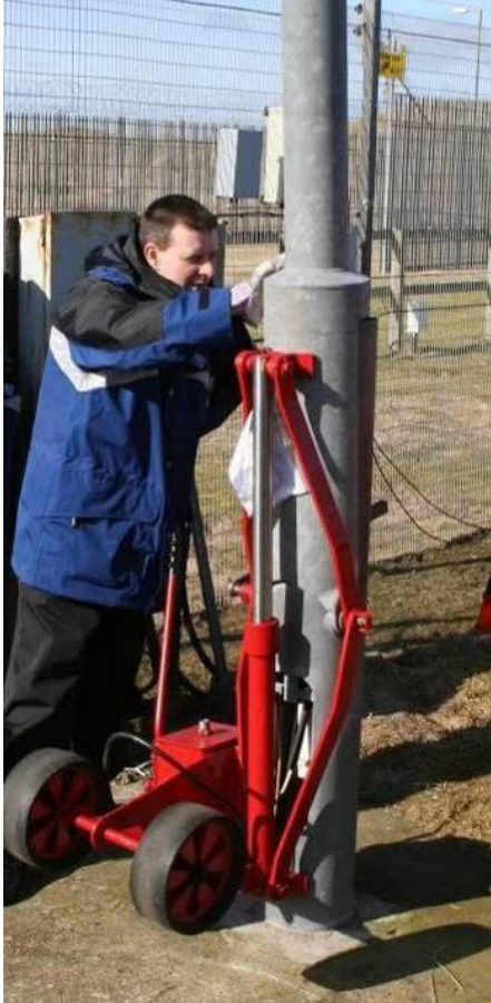
Demonstrating a one-man column lowering tool
